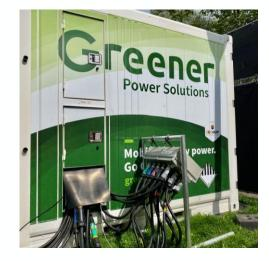
**Type 3; Capacity:** 225 kVA / 281-561 kWh
